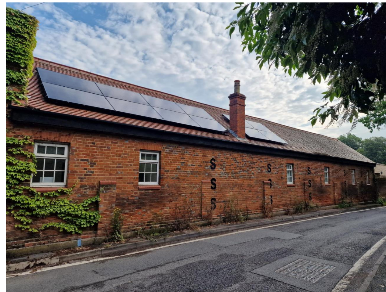
PV panels on Braywick Nature Centre
