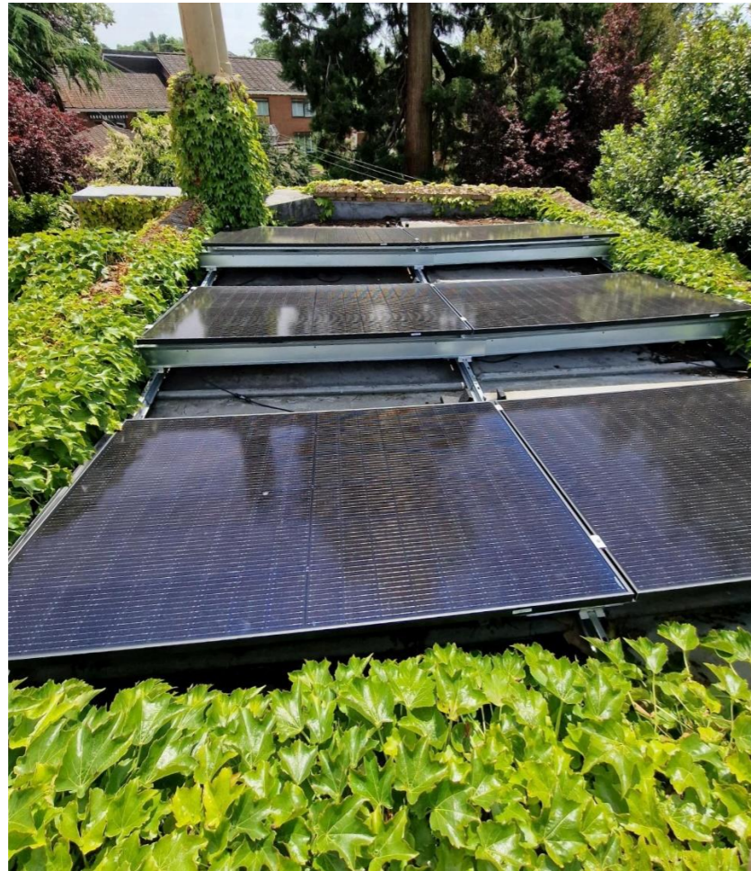
Bio-solar roof on Braywick Nature Centre
